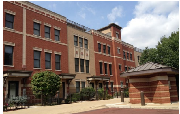
The neighborhood is home to a wide variety of housing types, from Atrium Village to modern townhomes such as River West.
