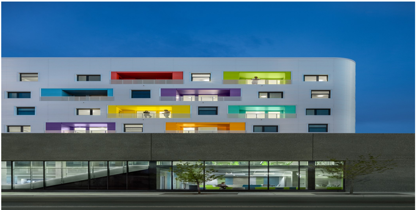
A view of the Independence Apartments and Independence Branch Library in the Irving Park community designed by John Ronan Architects
