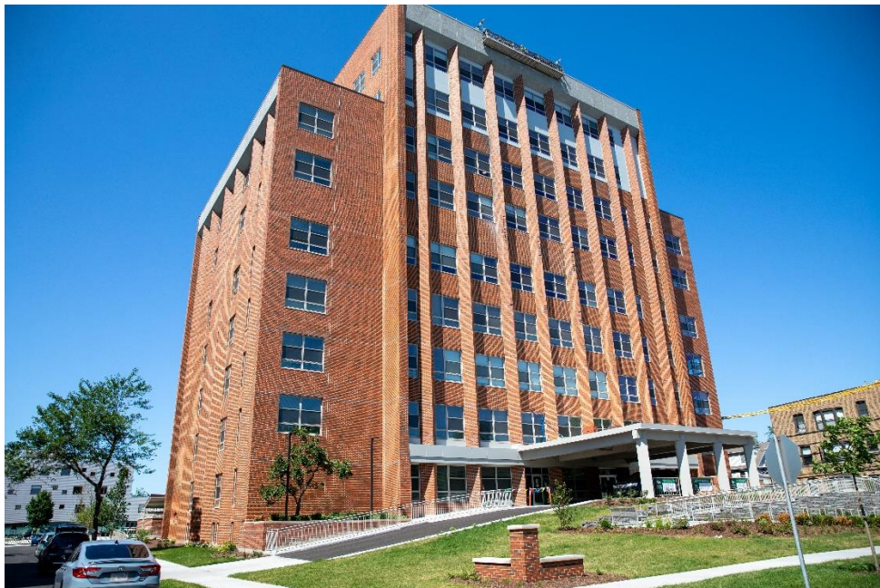
Ravenswood Senior Living is a public private partnership that combines affordable independent living with supportive living in one building, the first of its kind in Illinois.
