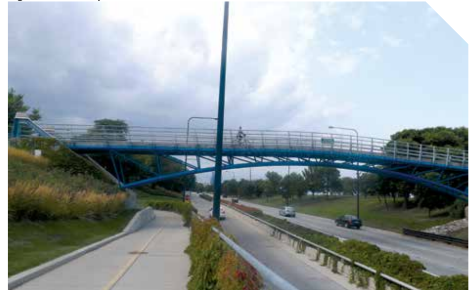
Figure 2.10. Overpass on 47th Street and Lake Shore Drive
