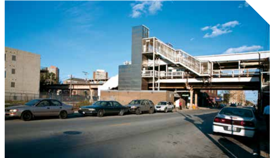
Figure 5.2. Parking near 43rd Street CTA station
